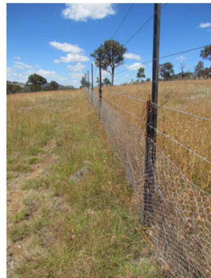
**Figure 8.** A kangaroo exclusion fence added to an existing cattle fence. The contrast between outside (left) and inside (right) in terms of grass growth can clearly be seen. The design was developed by ACT Parks and Conservation staff (see Supplementary Information, Data S1 for diagrams). (Photograph by Jenny Newport).
